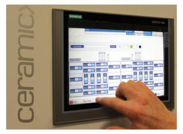
Touch screen HMI interfaces with the complete control system and provides the user with a graphic based visualisation of the process.
